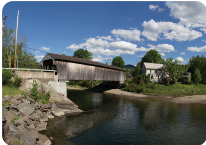
Village Covered Bridge Town of Waitsfield, VT
