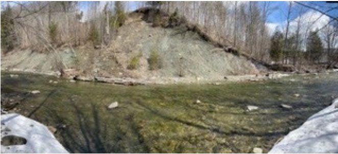
Landslide on Mill Brook at town boundary
