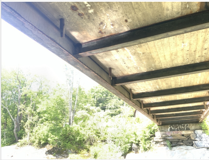
Floor beams at girder 1 from abutment 1
