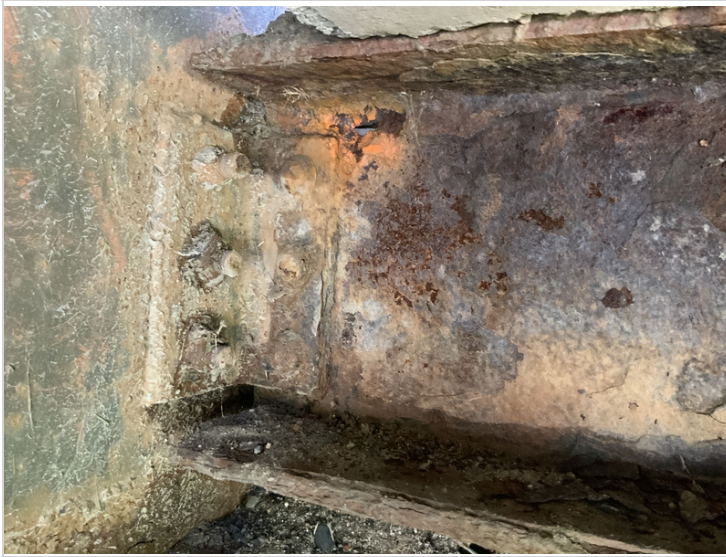
Floor beam 0 at girder 2
