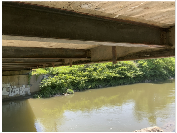
Floor beam ends at girder 1 from abutment 2
