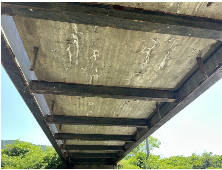
Deck and superstructure from abutment 2
