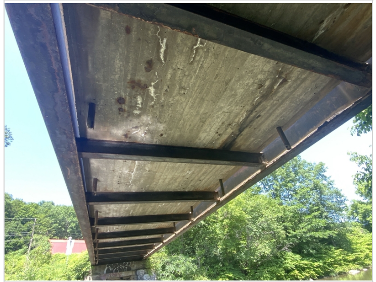
Soffit, superstructure and drains
