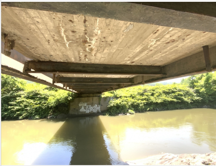
Floor beams from abutment 2
