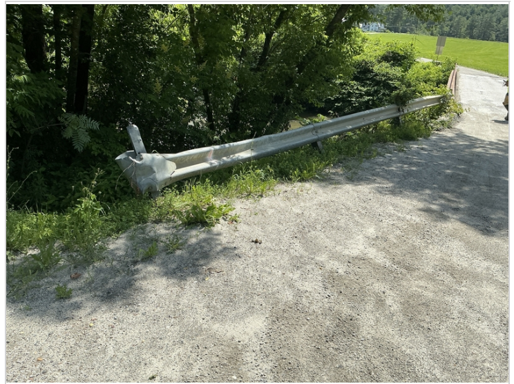
Approach rail and rail downstream abutment 2
