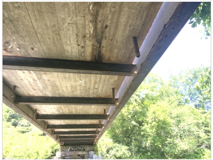
Floor beams at girder 2 from abutment 1
