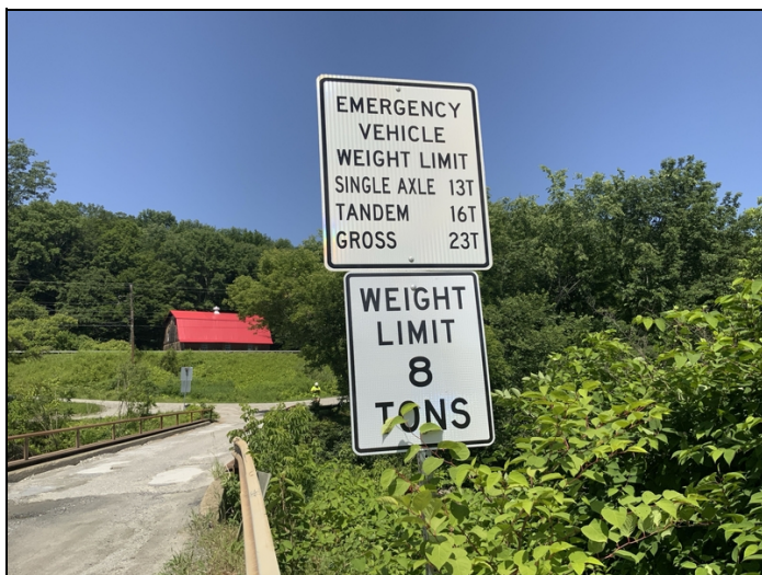
Abutment 1 EV sign
