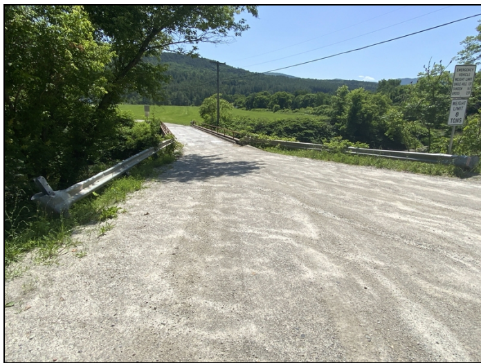
Abutment 2 approach rails
