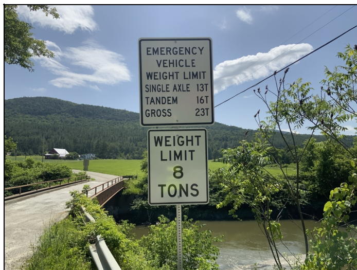
Abutment 2 EV sign
