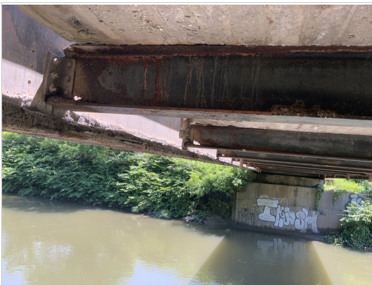
Floor beam ends at girder 2 from abutment 2
