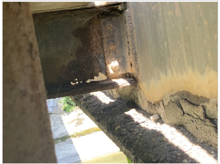
Floor beam 1 at girder 2
