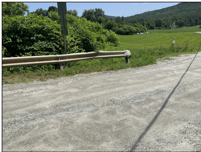
Abutment 1 downstream approach rail.
