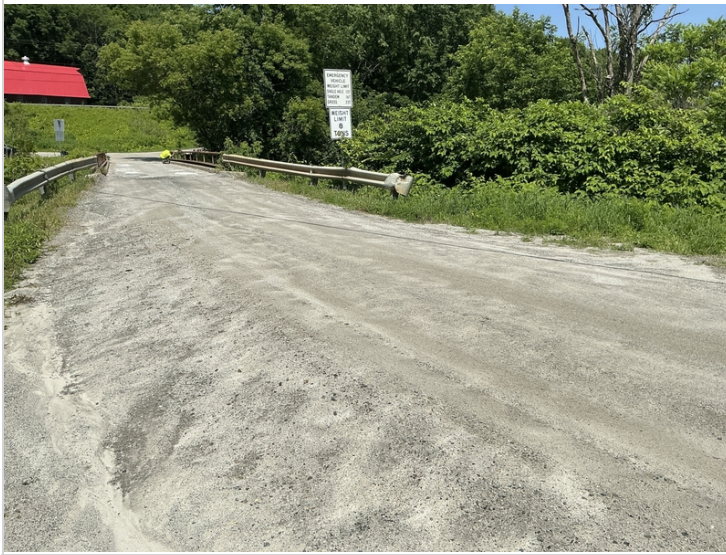
Approach rail and rail downstream abutment 1
