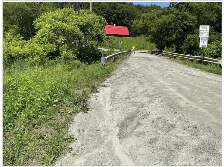
Approach rail and rail upstream abutment 1
