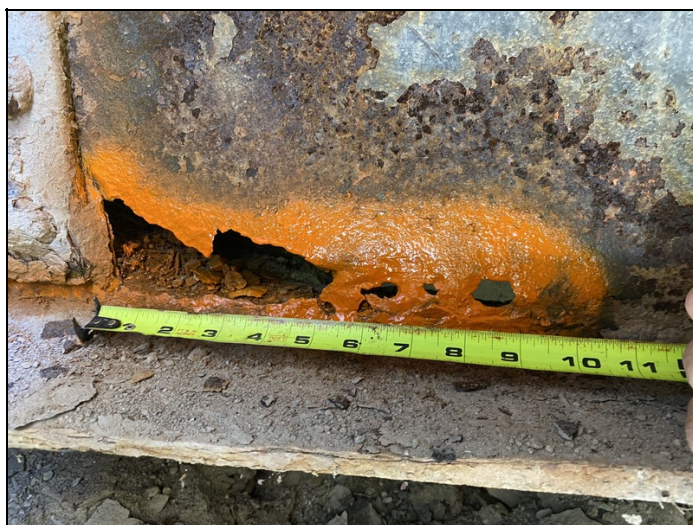
Floorbeam #9 at Girder #1
