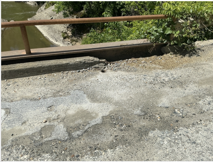
Curb upstream abutment 2
