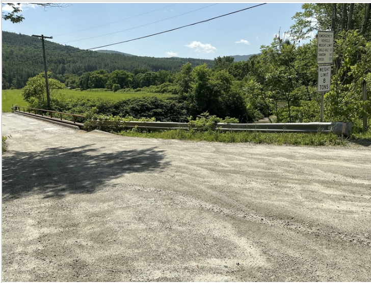
Approach rail and rail upstream abutment 2
