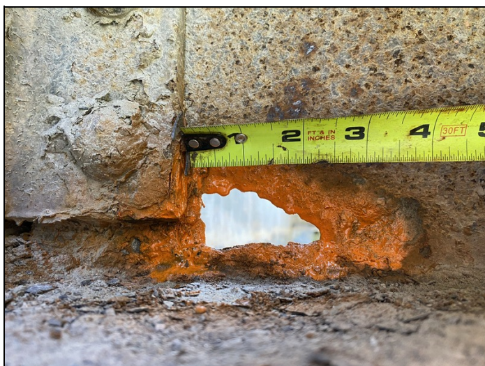
Floorbeam #6 at Girder #2
