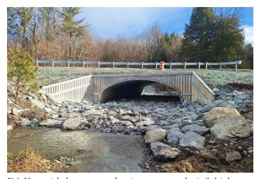
D&K provided survey, evaluation, structural, civil, highway, geotechnical, and water resources engineering, permitting assistance, bid phase services, and construction phase assistance for the replacement of a short-span, municipally owned culvert carrying a low-volume town highway over Judevine Brook. The existing structure was a 11-ft by 7-ft corrugated metal plate pipe culvert. The new bridge is a 28-ft
