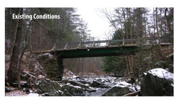
D&K completed a bridge study for the replacement of Bridge No. 080/120 on Archertown Road over Jacobs Brook. The project includes an alternatives evaluation and recommendations to replace the existing bridge, permit application assistance, preparation of final engineering plans and specifications, assisting the Town during the bid phase, and providing the Town with construction phase services.
