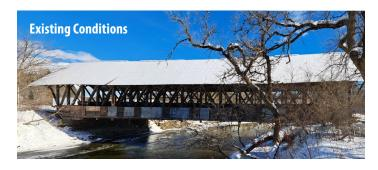
D&K is providing inspection, evaluation, and rehabilitation design of the Sanborn (Centre) Covered Bridge. The bridge provides pedestrian and snowmobile access over the Passumpsic River and is one of three Paddleford Truss-supported covered bridges of this type remaining in Vermont. The project is located within a floodplain, so significant hydrologic and hydraulic evaluations were required.
